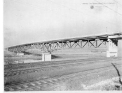
This view of the 7th Street Bridge shows the Santa Fe Railroad tracks, the Kaw River and the structural work of the bridge.
